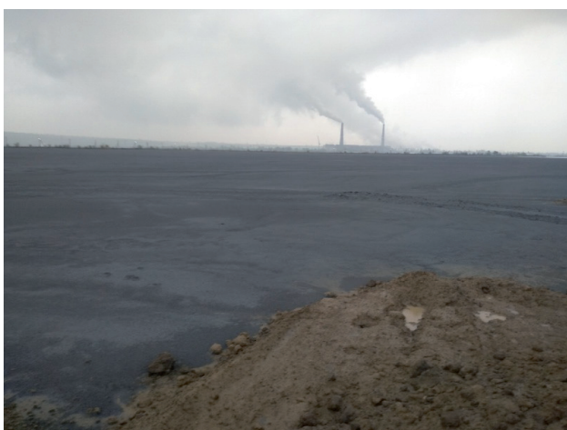
Fig.1. Aluminosilicate microspheres in the form of a “foam layer” on the surface of the ash dump. Almaty, Kazakhstan.
