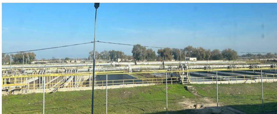
Figure 3 – Aerotanks for biological water purification of the Almaty Su enterprise using activated sludge
